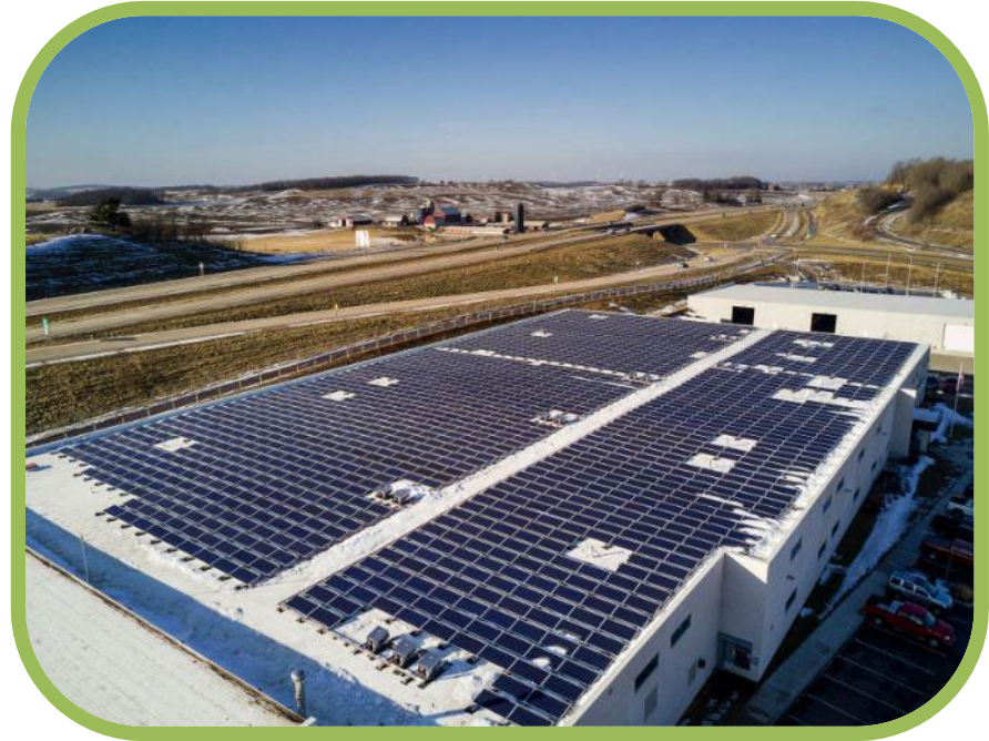
The roof of the Municipal Operations Center (MOC) in the City of Middleton is home to more than 1,700 solar panels as part of MGE's Shared Solar pilot project. This partnership between MGE and the City delivers 500-kilowatts (kW) of locally generated solar energy directly to MGE's community grid. Image source: MGE Energy
